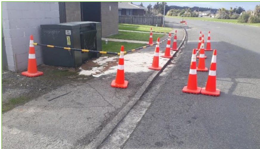
Figure 2: A local industrial site with its used oil receptacle and obvious hydrocarbon staining on the ground around the bottom of the tank.
