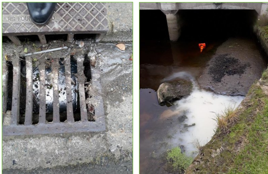
Figure 4: The results of a local contractor washing out his spray gun in a nearby stormwater sump.
