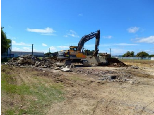
Softball Building Demolished December 2021
