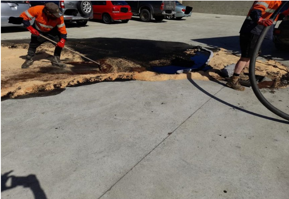
Figure 5: Clean-up of waste oil that has been spilled to stormwater at local industrial site
